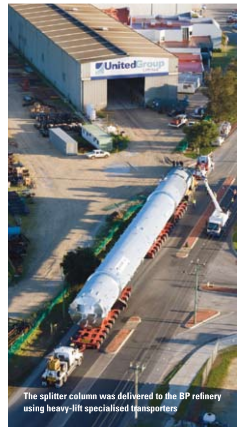
Beneath its shiny exterior more than 200 tonnes of XLERPLATE® steel went into the fabrication of the naphtha splitter
